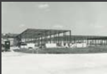
Construction of the Foley, Inc. Facility Piscataway, New Jersey - 1966
