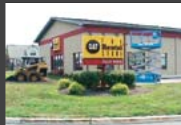
Foley Rents Facility Monroe, New Jersey - 2007
