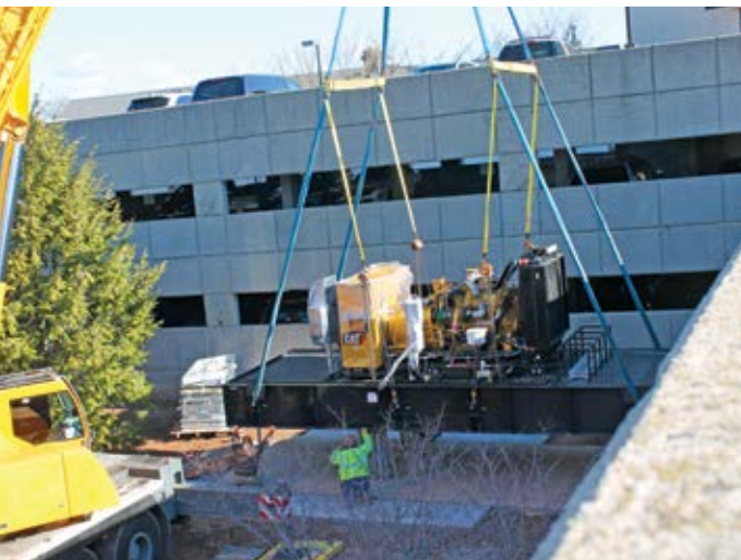
(L) A Cat C27 generator set is placed on a pad behind the City of Linden parking structure. (M) The genset enclosure is lowered into position. (R) Finished product blends in with surroundings.
