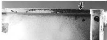
Illustration 76 g06344262 Erosion damage to the top land surface.
