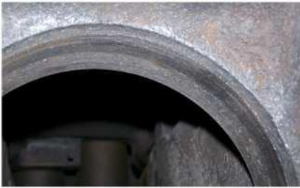
Illustration 117 g06238803 Erosion in the lower cylinder bore
