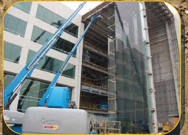
County Glass & Metal of Hackensack, NJ is putting these Genie boom lifts to work on a jobsite in Hanover, NJ. The S85 and S125 are being used to create glass walls for an atrium on the building pictured.
