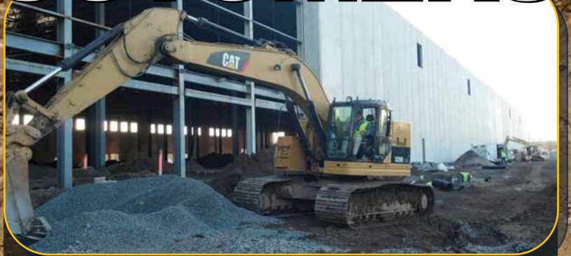
Charlie Dandeneneau, of Concrete Construction Corp., is operating his new 328 Hydraulic Excavator to back-fill on the company's jobsite in Carteret, NJ where they are constructing an underground detention basin to collect storm water from a large warehouse and parking lots.
