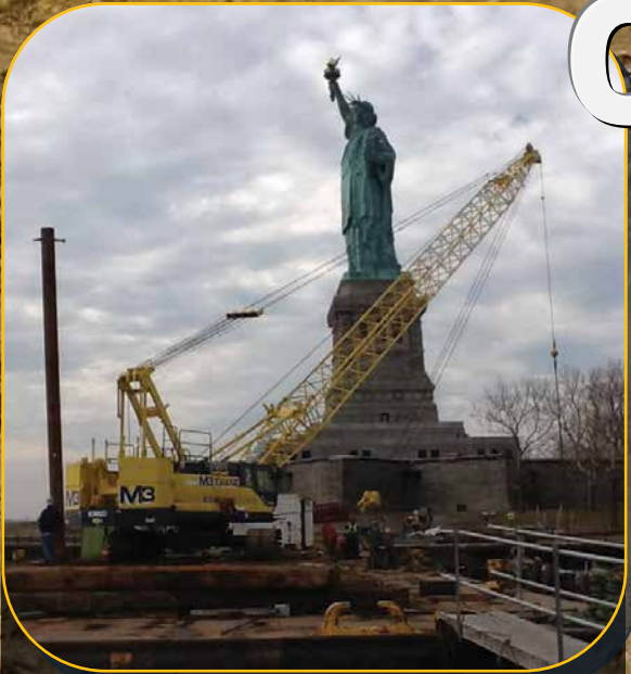
M-3 Crane works on Ellis Island alongside Lady Liberty herself, using their newly purchased CK-1100G Kobelco Crane.
