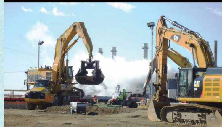
Barbella-Kollasch is using a 5110 B HRD (high reach demolition) machine to dredge the old NASCAR property on the Bayonne side of the Goethals Bridge.
