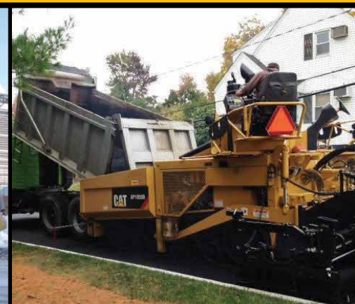
S. Brothers of Manalapan, N.J., repairs damaged asphalt by paving side-streets with their AP 1055 D.
