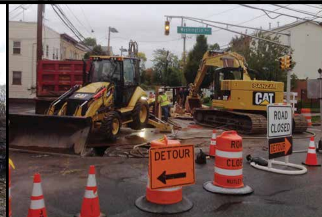
Joseph M. Sanzari Inc. performs emergency sewer repairs with new 420 F and 321 DLCR machines.
