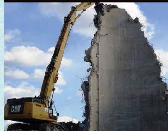
Control Services LLC., of Jersey City, N.J., added a 349 E high-reach excavator to their fleet this year to perform jobs like taking down this building in Avenel.
