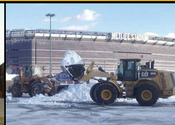
After the brutal winter in N.J., J. Fletcher Creamer works to clear out some of the MetLife Stadium parking lot to make way for Giants and Jets fans.
