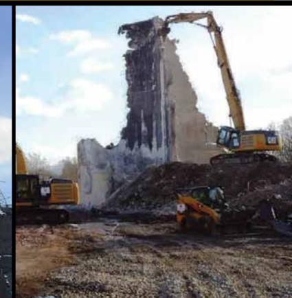
Control Services LLC., of Jersey City, N.J., added a 349 E high-reach excavator to their fleet this year to perform jobs like taking down this building in Avenel.
