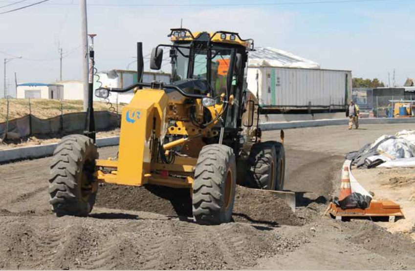
TOP Union Paving and its Cat machines will lay down a Route 35 roadbed that is much stronger than the previous surface.
