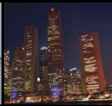
Building Load Test
