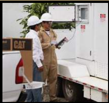
Load Bank Testing
